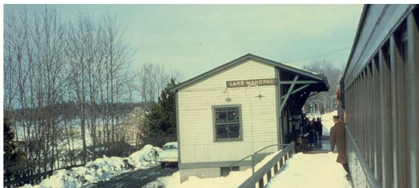
Lake Mahopac - Thompson House Station
